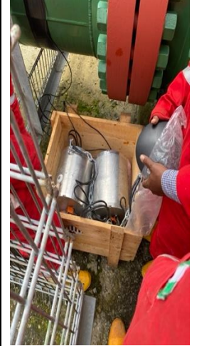
Installation of the nodes on site.
