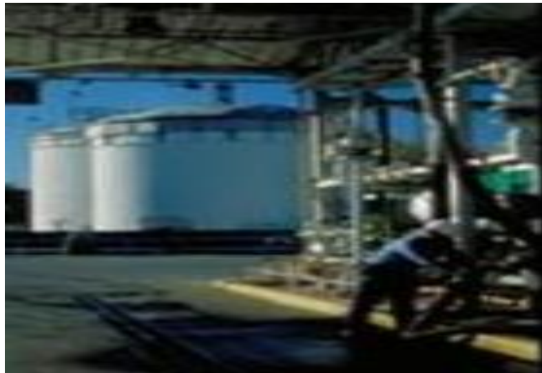
Storage Tanks Integrity inspection and corrosion monitoring
