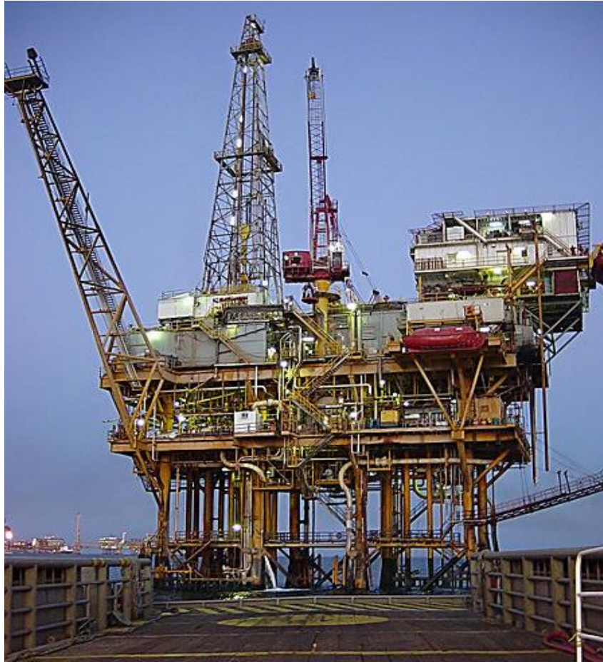
Oil Platform integrity inspection and vibration monitoring
