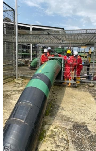
Complete installation of Sensors on site - FRM
