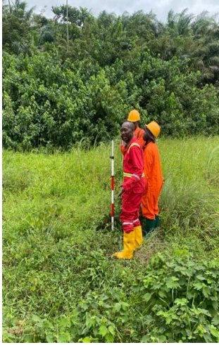
Site Inspection for Nodes Installation at FRM – Forcados.
